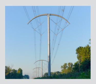
AEP Ohio chose BOLD for the project because of the aesthetic and environmentally friendly benefits, and the superior electrical characteristics the design provides. The towers will be shorter than alternative traditional structures would be, helping them to blend with the landscape. Two circuits will replace the original single circuit without additional rights-of-way required.
